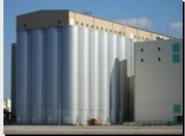
Raw grain silos
